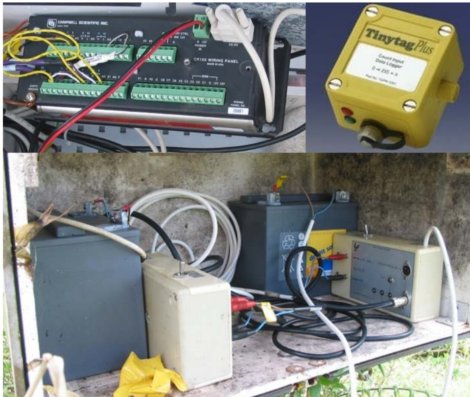
Figure II.4. The CR10X-datalogger of Campbell Scientific (top left), the Tinytag single channel puls datalogger (top right) and power supply by batteries charged in turn by solar panels (bottom).
