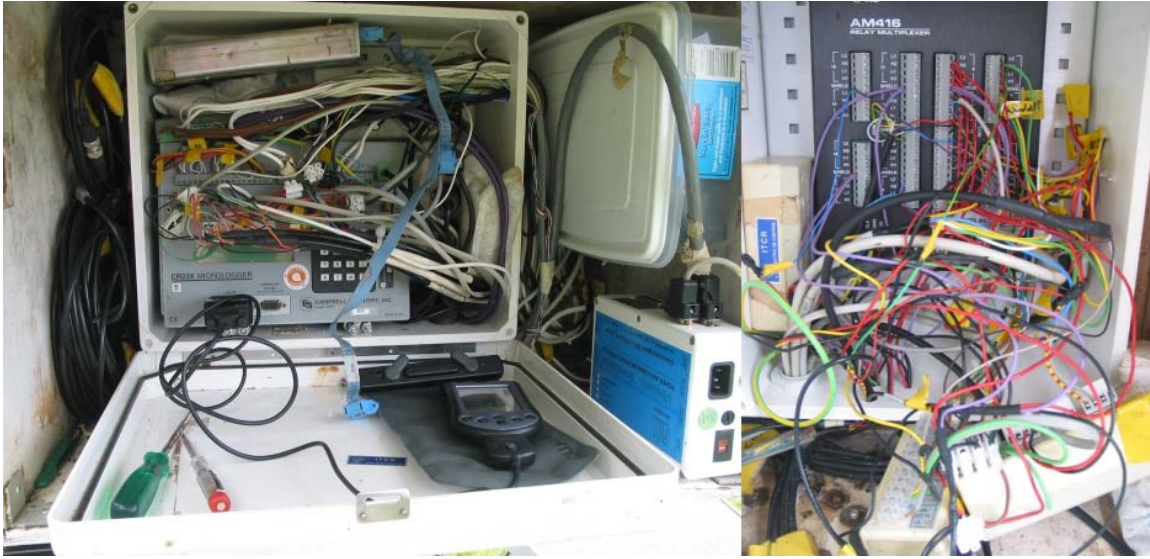
Figure II.5. CR23X-datalogger for automatic data recording (left). An AM416 relay multiplexer is used to increase the number of input channels to the data logger (right).
